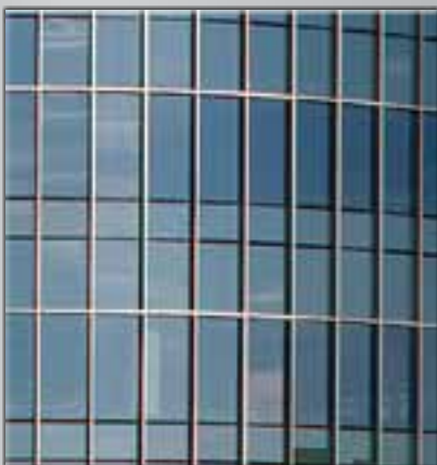
Building facade glazed curtain wall
